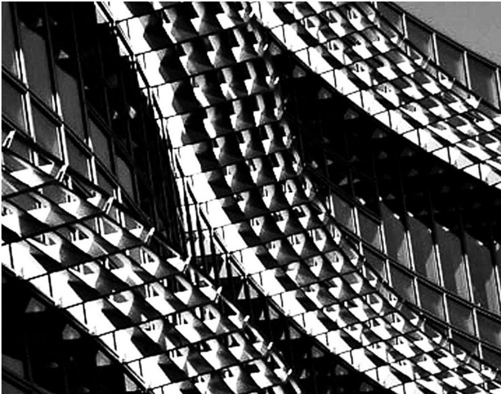
FOUND MATH: CURVED SURFACES AND SPATIAL TESSELLATIONS AROUND ON THE ALCOA CORPORATE CENTER ON PITTSBURGH'S NORTH SHORE. PHOTO COURTESY OF ALESSANDRO ARSIE (UNIVERSITY OF TOLEDO)
