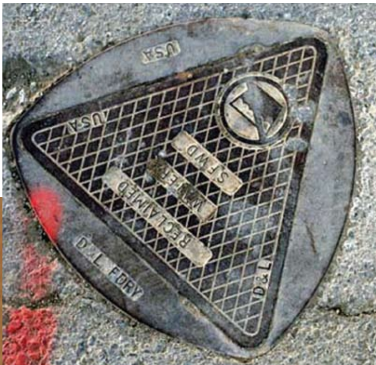
Above: Because Reuleaux triangles have a constant width, this triangular manhole cover in San Francisco would be just as unlikely as circular ones to fall through the opening. Photo by Owen Byrne.
